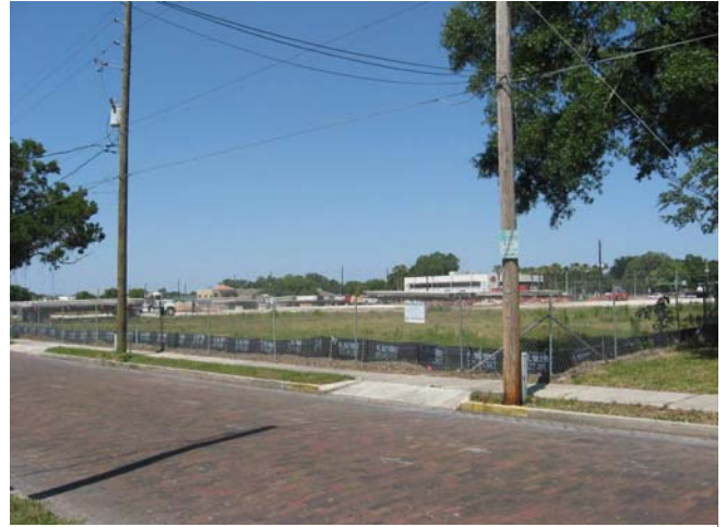
Mills Park Development site located to the northeast of the subject site.
