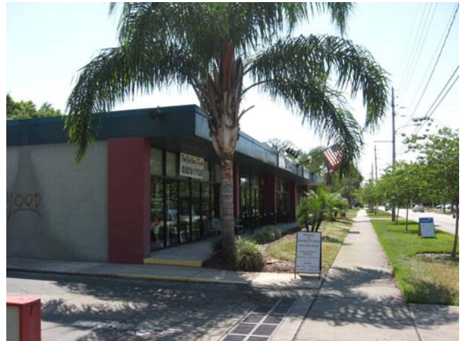
Exiting one story commercial building to the south of the subject site along Virginia Drive.
